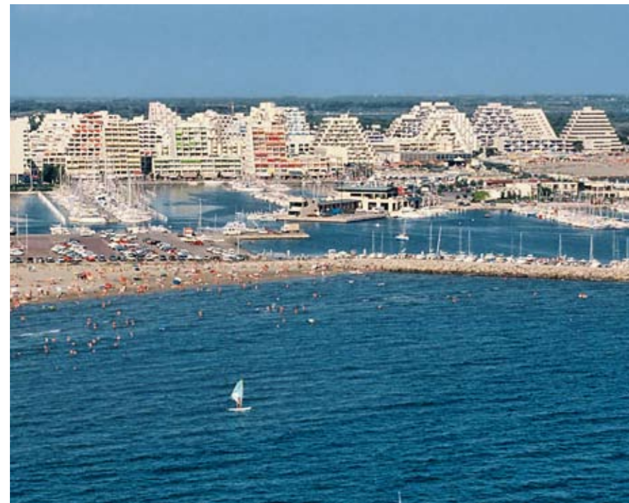
Urban sprawl and waste of resources – the building boom in popular coastal holiday resorts deteriorates the climate balance. © Michel Gunther / WWF-Canon
